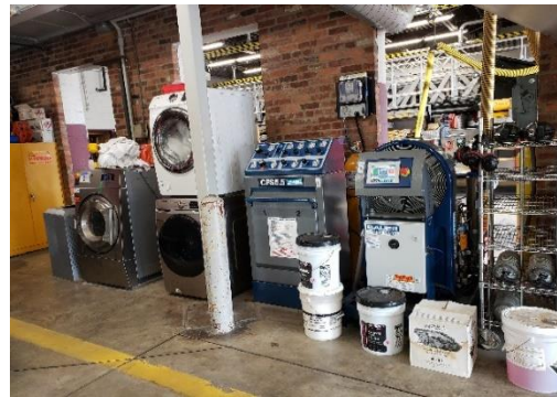
Air Compressor and Cleaning Supply Storage
